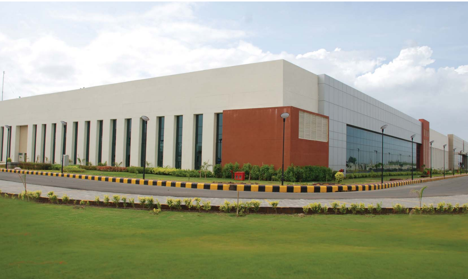
Switchgear Factory, Baroda
